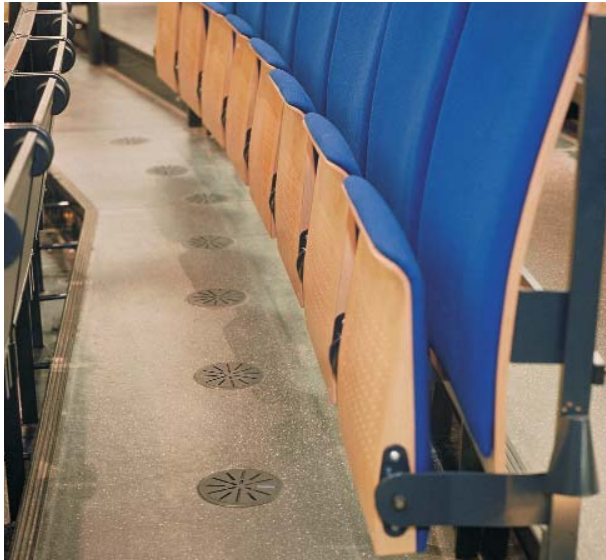
Floor displacement outlet, type Q-B-DN 200, with clamp insert in floor tile
