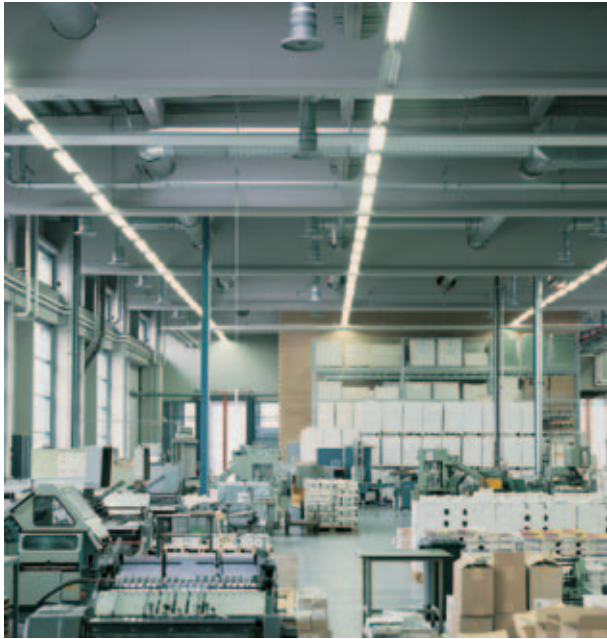
Fig. 7: Radial displacement outlet in a printing shop
