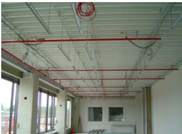
Fig. 6: For sail suspension, the fastening crossbars are suspended from the ceiling using threaded rods and their position is adjusted in height and alignment
