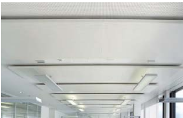
Fig. 7: Installed multifunction sails
